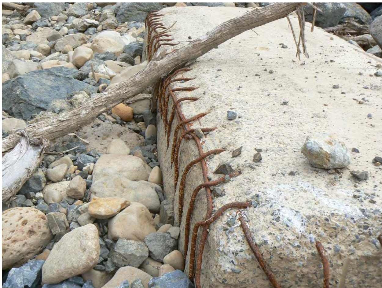
Photo 7 – A 7 tonne sill block carried 150m
