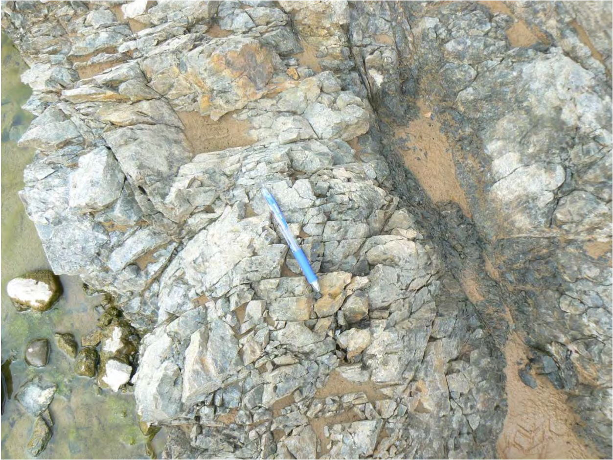
Photo 10 – Closely Fractured Rock Less Resistant to Scour
