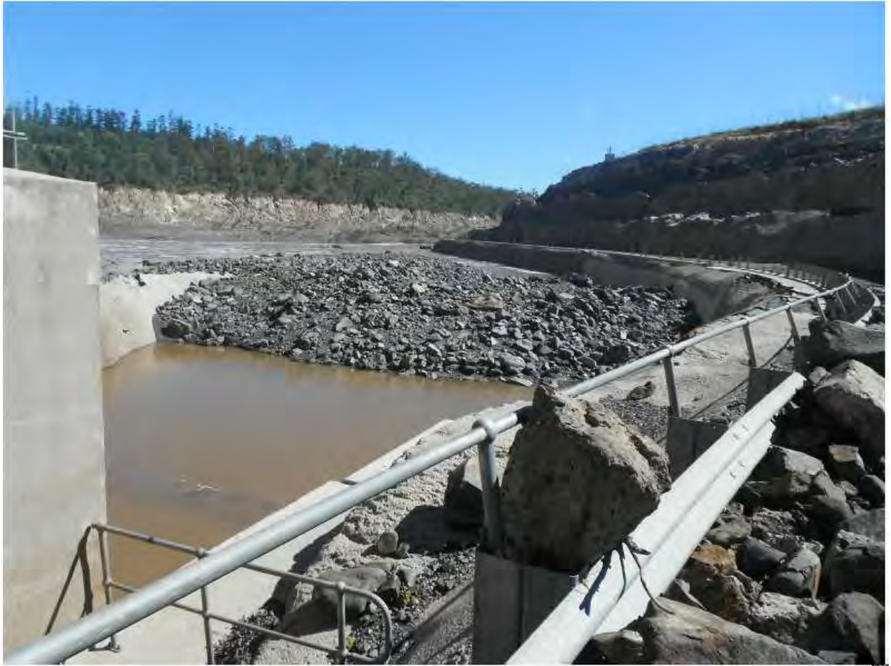
Figure 6 – Rock and Gravel in the Near Vicinity of the Dissipator
