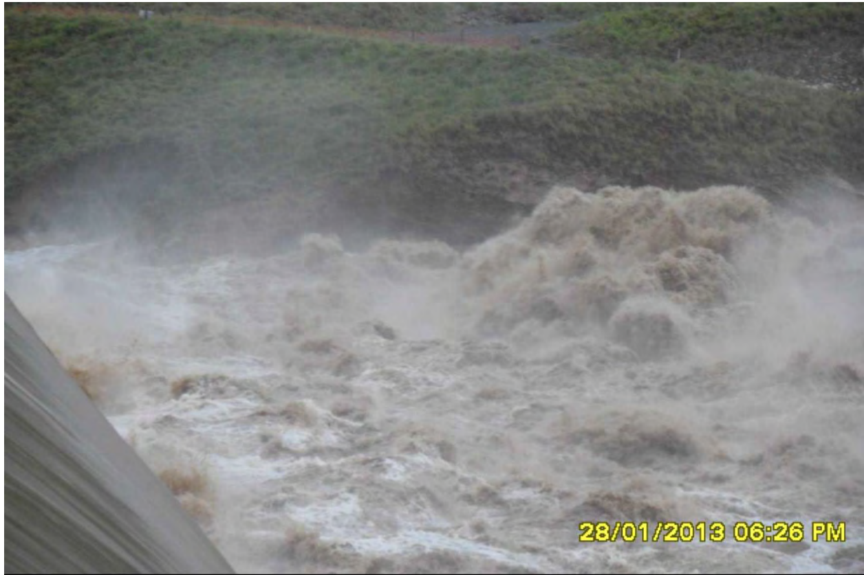
Figure 2 – Turbulent Flow at the Left End of the Spillway
