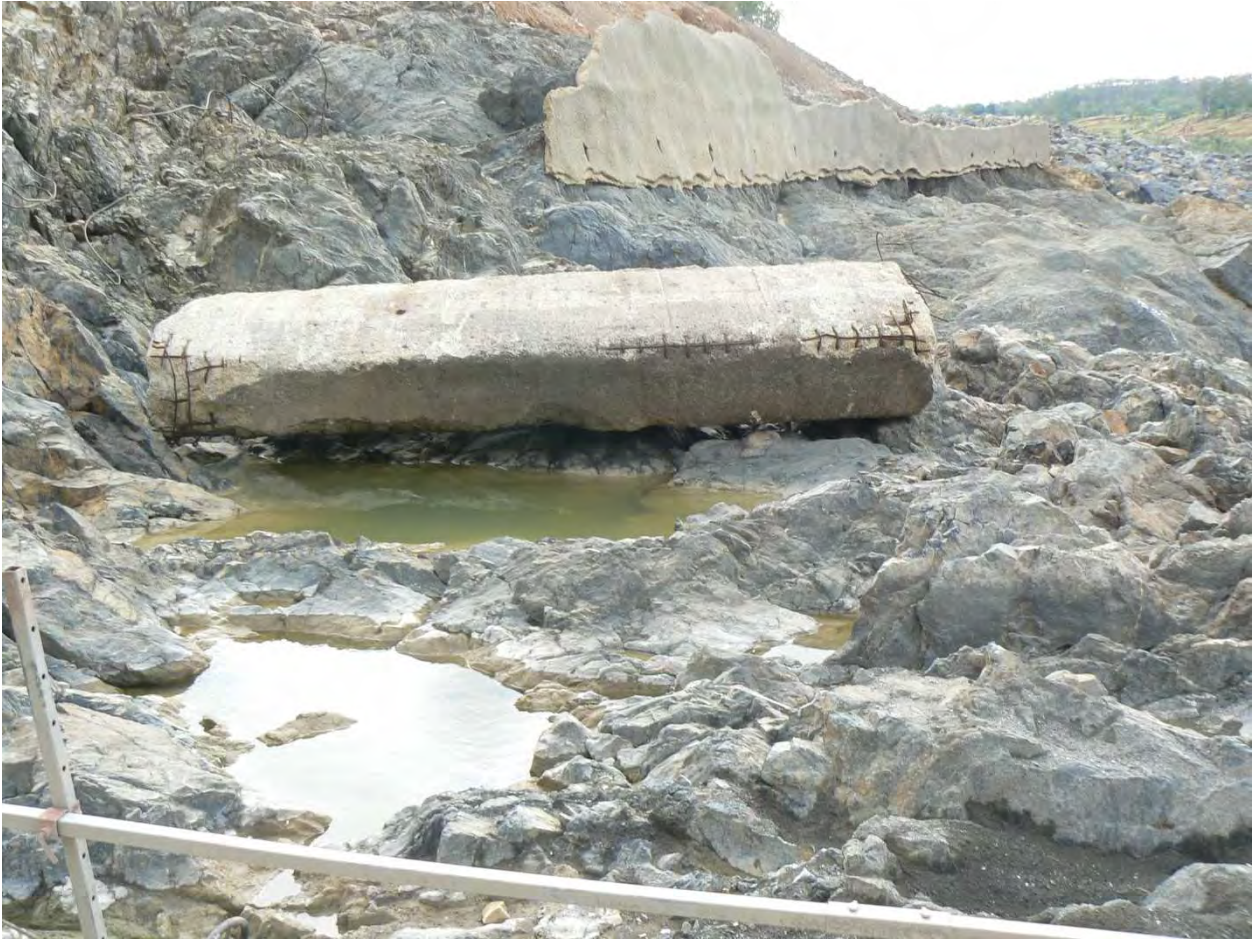
Photo 3 – Sill Block at Base of Left Abutment
